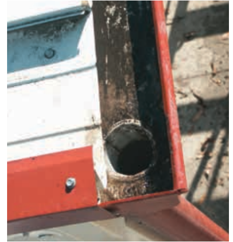
3) When litter is removed, the layer of hardened dirt is revealed below.
