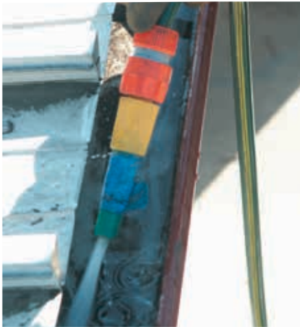
4) Rinse the gutter with water to soften and break up the dirt.
