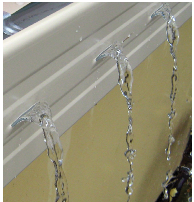
Typical overflow from slotted gutter.
