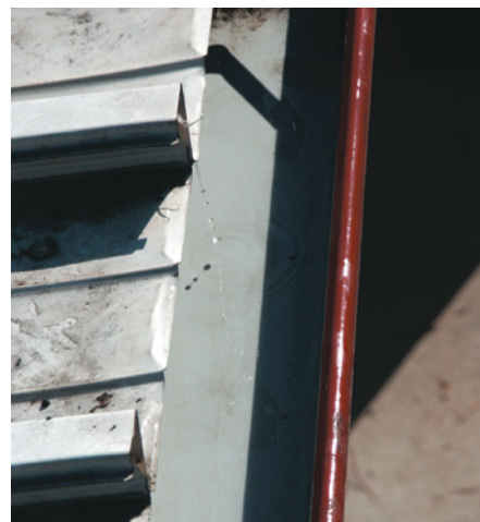
6) When the gutter has been cleaned, it should look like this.
