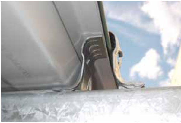
Figure 4b Position the 'S' clips over the male lapping rib of the cladding.
