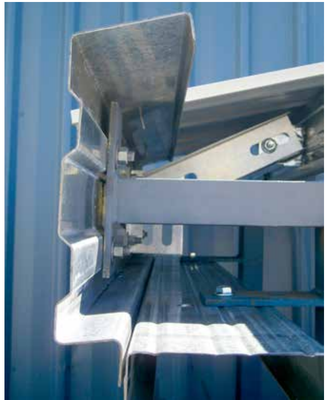
Fascia purlin shown mounted on a building
